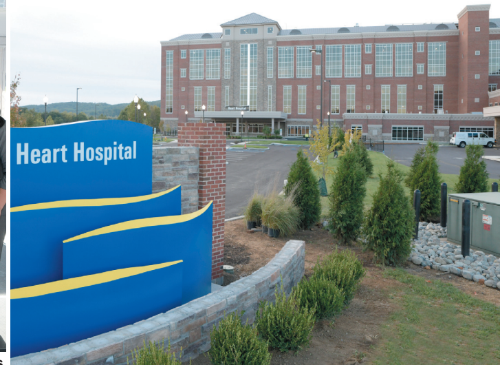
The Heart Hospital is the largest construction project in St. Luke's more than 150-year history, both in dollar figure ($252 million) and square footage, five-story, approximately 355,000-square-foot the upper floors stretches 330 feet — roughly the length of a football field
